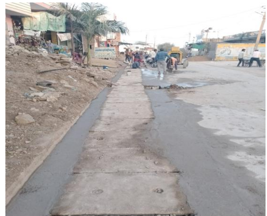
Drain work at Gadepan
