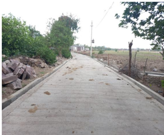
Cement Concrete Road in Gadepan
