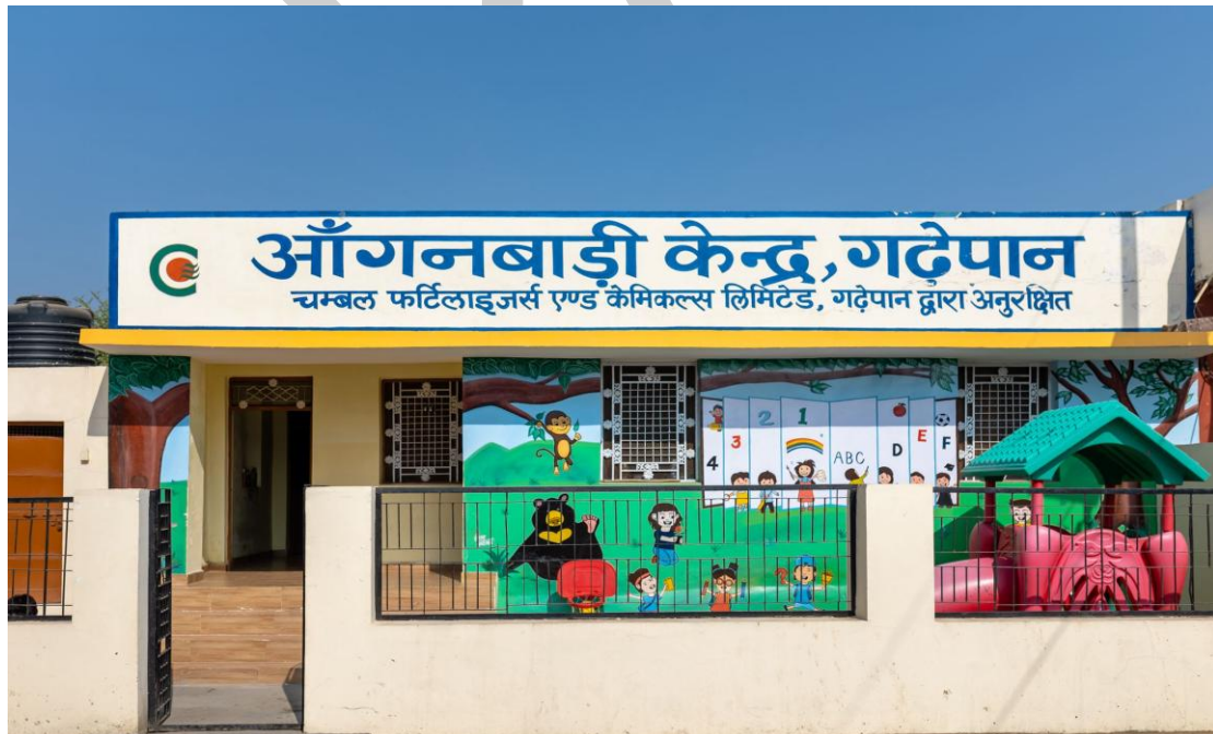
Figure 4: Anganwadi renovation under project Akshar
